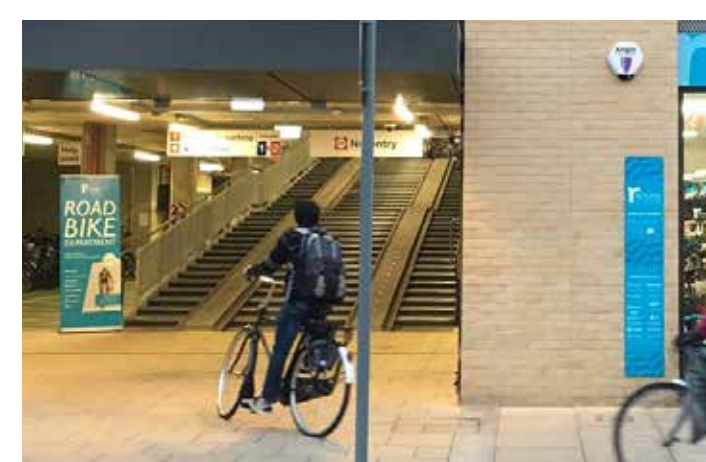
Cycle access to the basement will be via a ramp like at the station.
