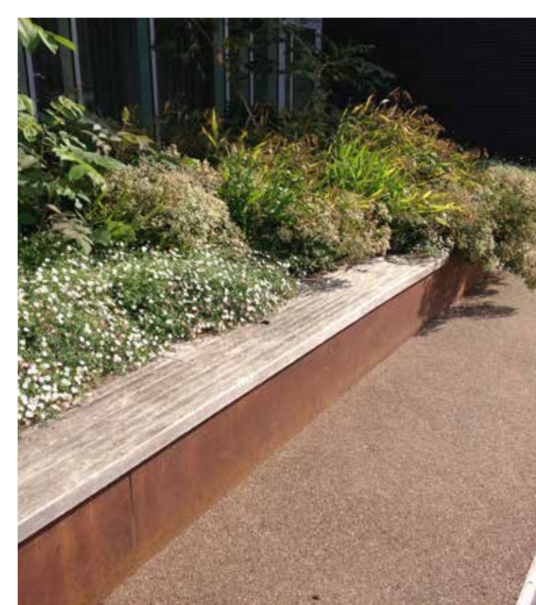
raised planting beds with timber seat tops
